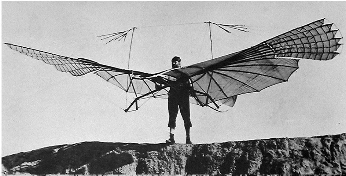
Fig. Some of Lilienthal's later designs show multiple leather-like wing tips. These were intended to flap, reproducing the action revealed in the high-speed photography of Morry and Maybridge.
